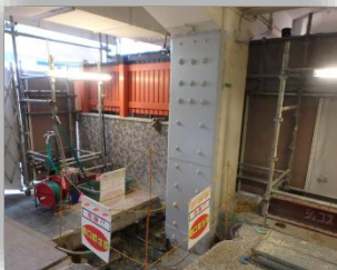
Example: Seismic reinforcement of columns and stations
