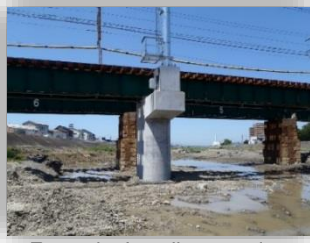
Example: Install measuring instruments on bridge piers
