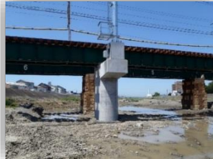
Example: Install measuring instruments on bridge piers
