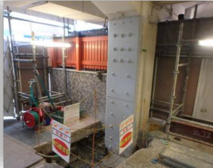
Example: Seismic reinforcement of columns and stations
