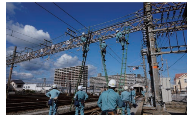
Restoration training by electrician staff
