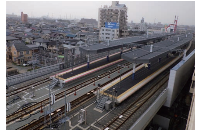
Continuous grade separation project in Takaishi City
