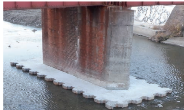
Countermeasure work to prevent the scour of a bridge over the Tsuda River
