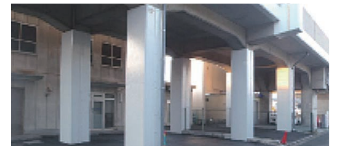
Reinforcement of overpass pillar earthquake resistance (by wrapping with steel sheets)
