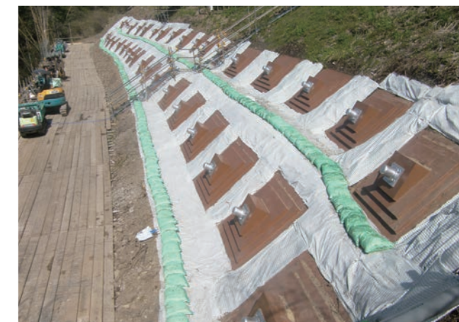
Two rows of anchor reinforcements installed on slope
