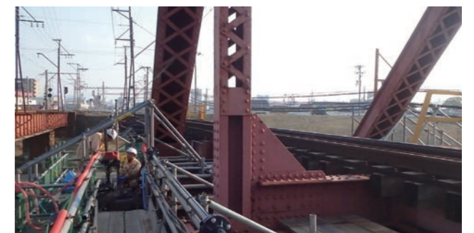
Reinforcement of Kinokawa Bridge piers on Nankai Line (incorporation of steel bars)
