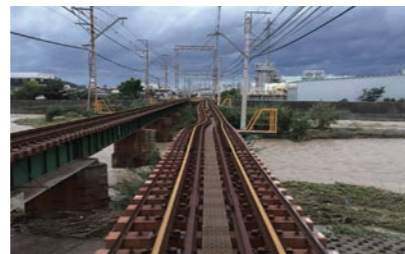
Outbound track with leaning bridge pier and bent rail
