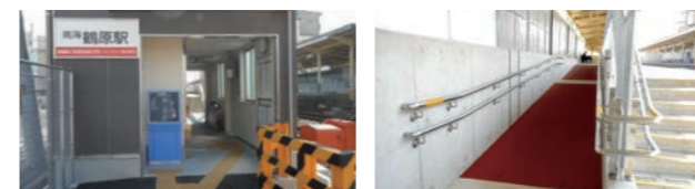
Slope installed and new east entrance added (Tsuruhara Station)
