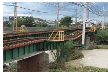
Outbound track with leaning bridge pier and bent rail
