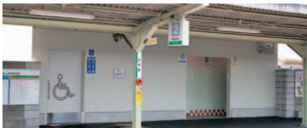
Toilet facilities at Sayama Station following barrier-free construction work
