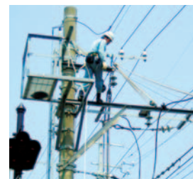
Work-site training on a feeder and a pole
