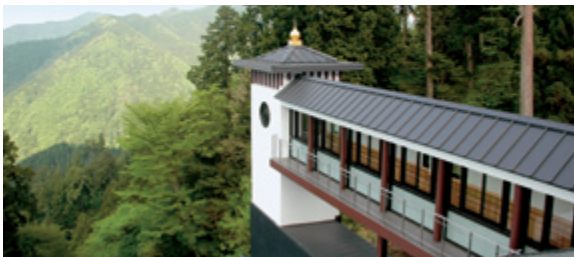
Elevator at Kōyasan Station
