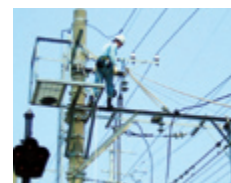
Work-site training on a feeder and a pole
