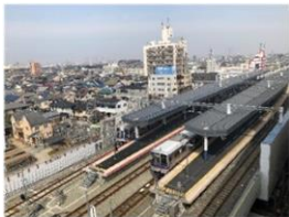
Continuous flyover roadway construction projects in Takaishi City
