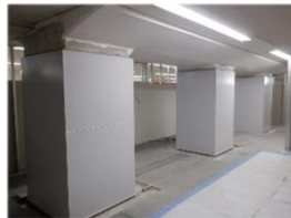
Seismic retrofit of Kishinosato-Tamade Station
