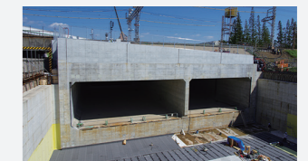
Construction of overpass between roads and railroads
