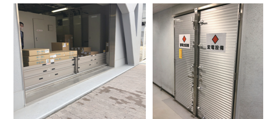
Tide embankment (left) and a watertight door (right) (Tamade General Office)
