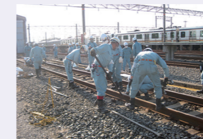
Restoration of railroad track facilities
