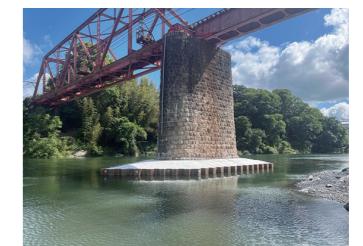
Scouring prevention measures (Kinokawa River Bridge, Koya Line)
