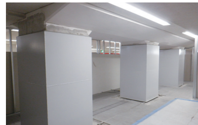
Kishinosato-Tamade Station seismic retrofitting
