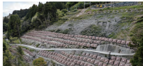
Construction to prevent landslides (within Kamikosawa Station)
